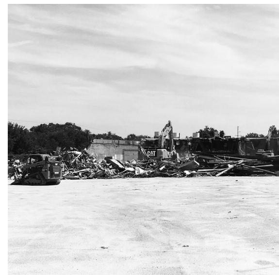
The former grocery store building was demolished in May 2018.
